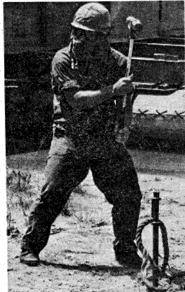
PVT William Johnson drives a supporting stake into the bank of Victory Pond to lash a portion of bridging equipment to the shore during tactical rafting and bridging operations.
